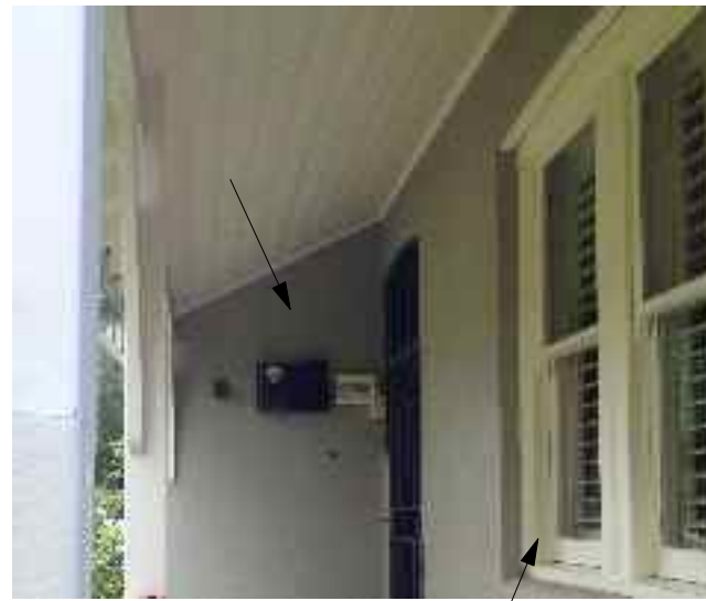
V-jointed lining boards, lining underside of veranda ceilings
