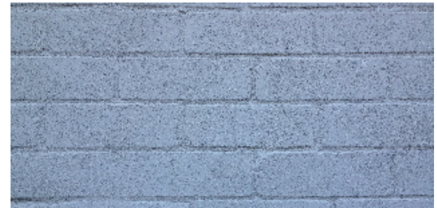
BAGGED BRICKWORK- To match existing external walls
