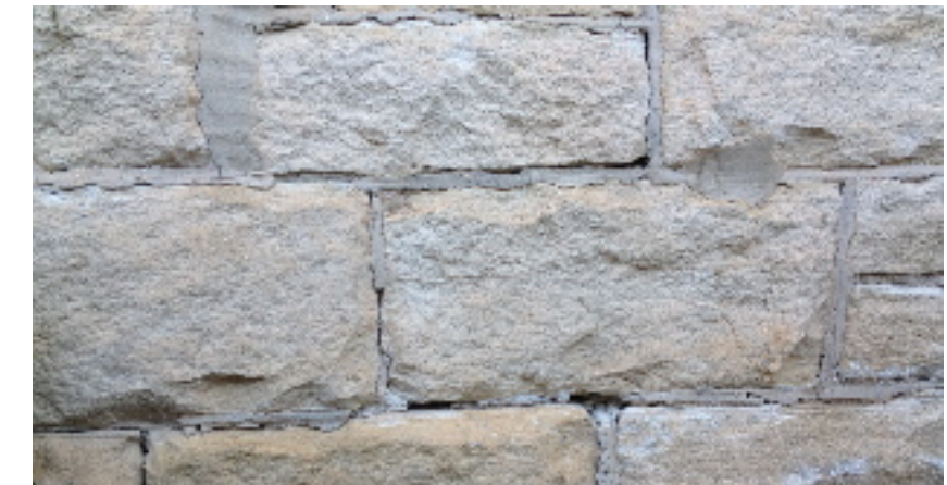
RE-USE EXISTING SANDSTONE- For subfloor walls below veranda & subfloor below entry.
