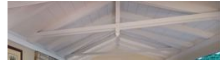
EXPOSED TIMBER TRUSS- to raked ceiling in proposed living room
